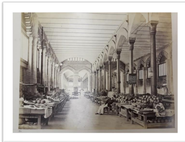
Figure 4.5 Interior of the Hogg Market, Calcutta, 1876 (Source: British Library, London)
