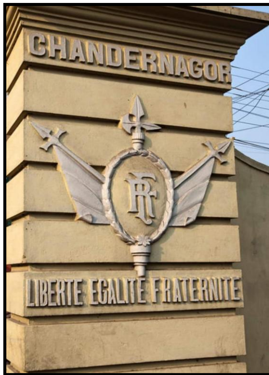
Picture- 4, The Barasat gate, located at Borobazar, Bhadeshwar, marks the border of Chandannagar (under the French regime) and Bhadeshwar (under the British regime). Personal collection, Chandannagar, 14.7.2021.
