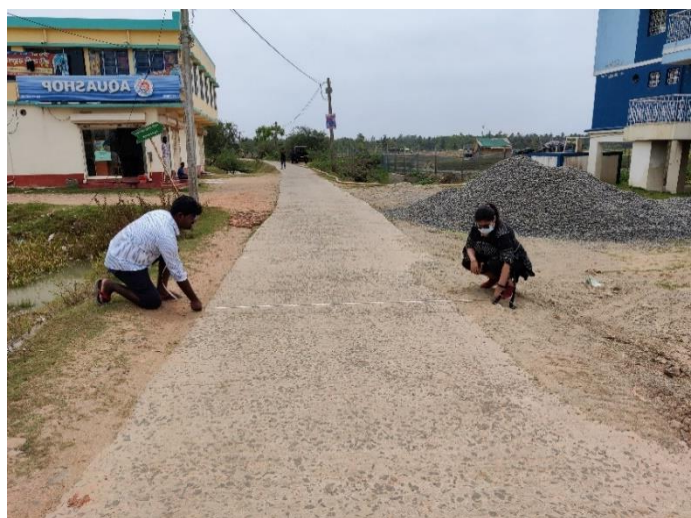
Figure 14: A concrete road in Deshapran block
