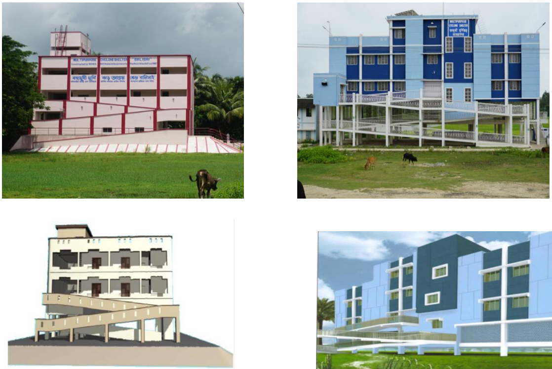
Figure 20: View of the MPCS constructed under PMNRF and NCRMP-II respectively, photographs taken by the author, May 2019. Graphical image Source: (GoI, 2006) and (Government of West Bengal, 2017)
