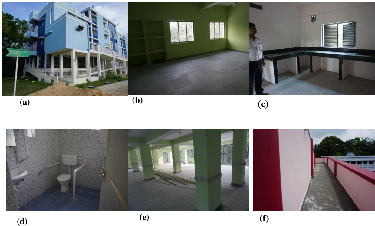
Figure 23: (a) view of the MPCS, (b) hall for people to take shelter, (c) kitchen, (d) toilet for specially abled person, (e) space for cattle, (f) ramp for easy entry into the MPCS. Photographs taken by author
