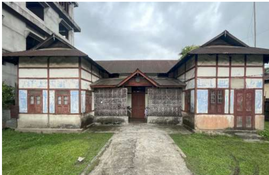
Figure 2.6: Moderate Sized Openings, Symmetrical Design, Simple Roof Structure etc in a Traditional Assam-Type House (Source: Author)
