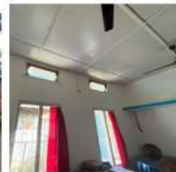
WALL AND CEILING
