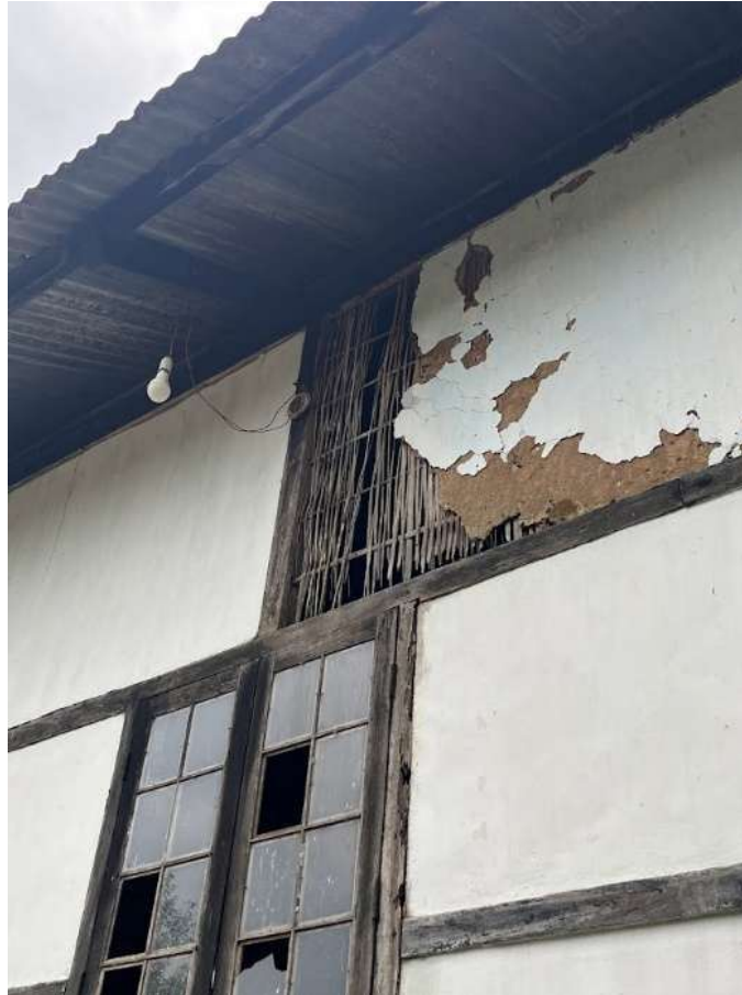
Figure 2.4: Visible Materials in a Partially Exposed Section of a Traditional Assam-Type House (Source: Author)
