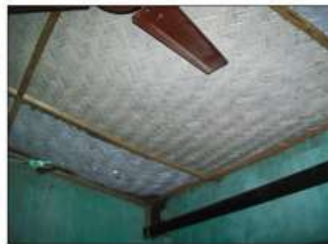
WALL AND CEILING
