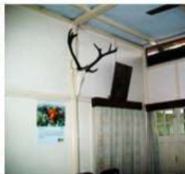
WALL AND CEILING
