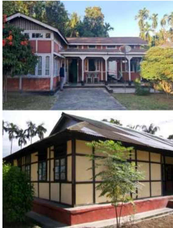
Figure 4.12: Traditional Assam-Type Houses in Warm and Humid Climatic Zone, Bilasipara, Assam (Source: Author)
