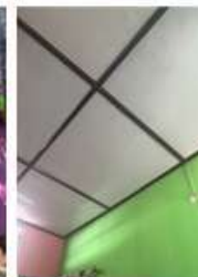
WALL AND CEILING
