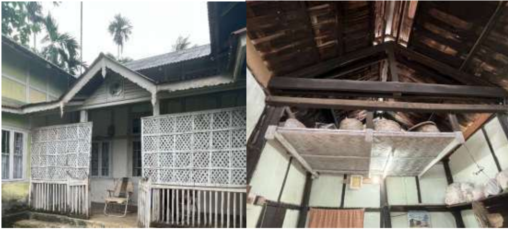
Figure 2.13: Example of a Bamboo Screen and Attic Storage Space in Traditional Assam-Type Houses (Source: Author)
