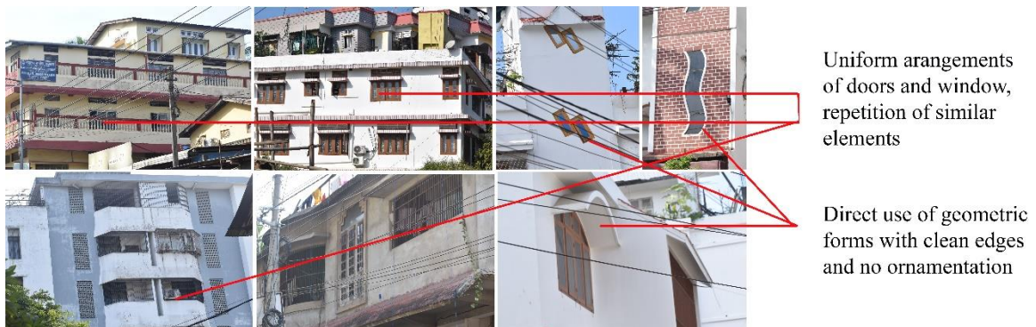
Fig. 5.9: Photographs of doors and windows of built forms of Hengrabari
