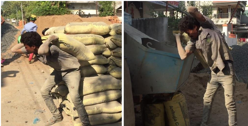
Figure (iii) Lifting, Transportation and unloading of cement sack
