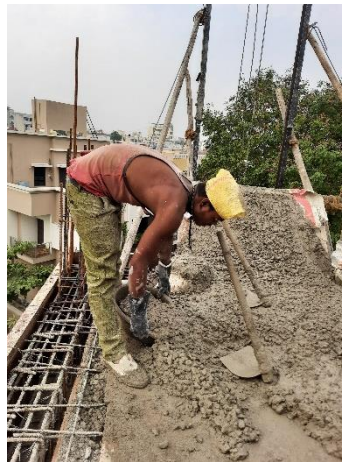
Figure (b): Lifting of Iron-Pan
