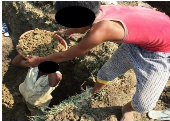
Figure (v): Outside labour receive Iron-pan from Inside labour (Job-5)
