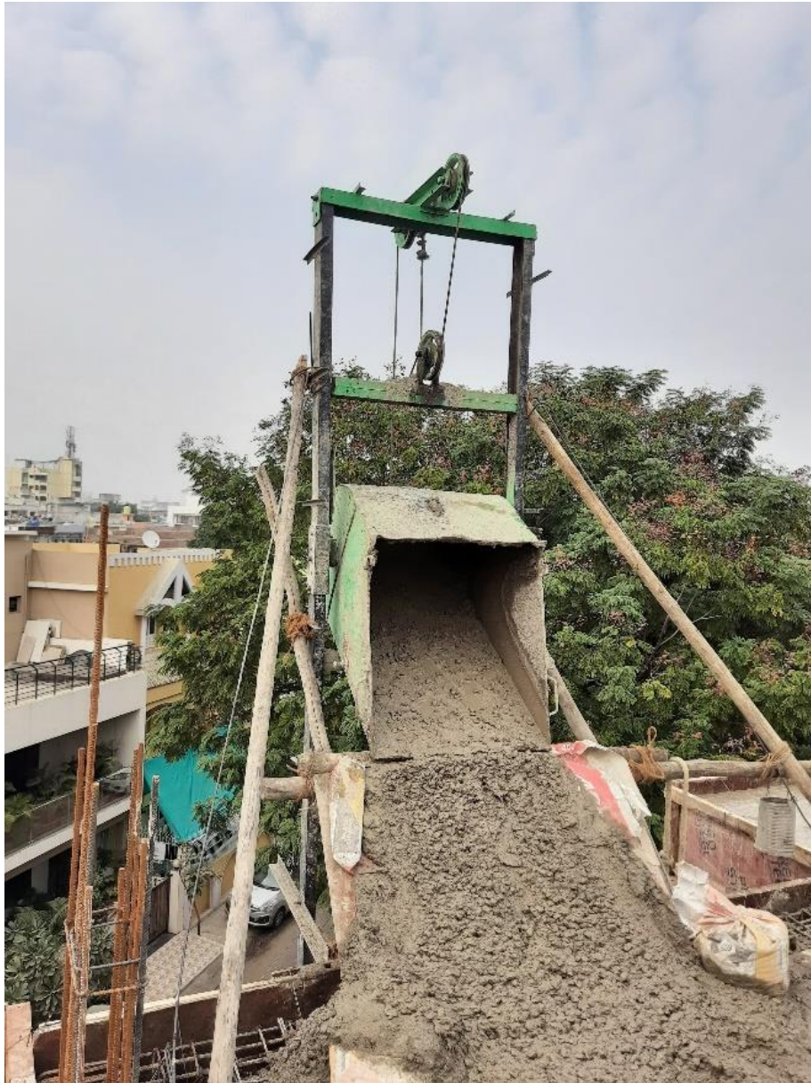
Figure (i) Figure of real time elevator with hopper releasing concrete on floor (unloading of concrete mixture)
