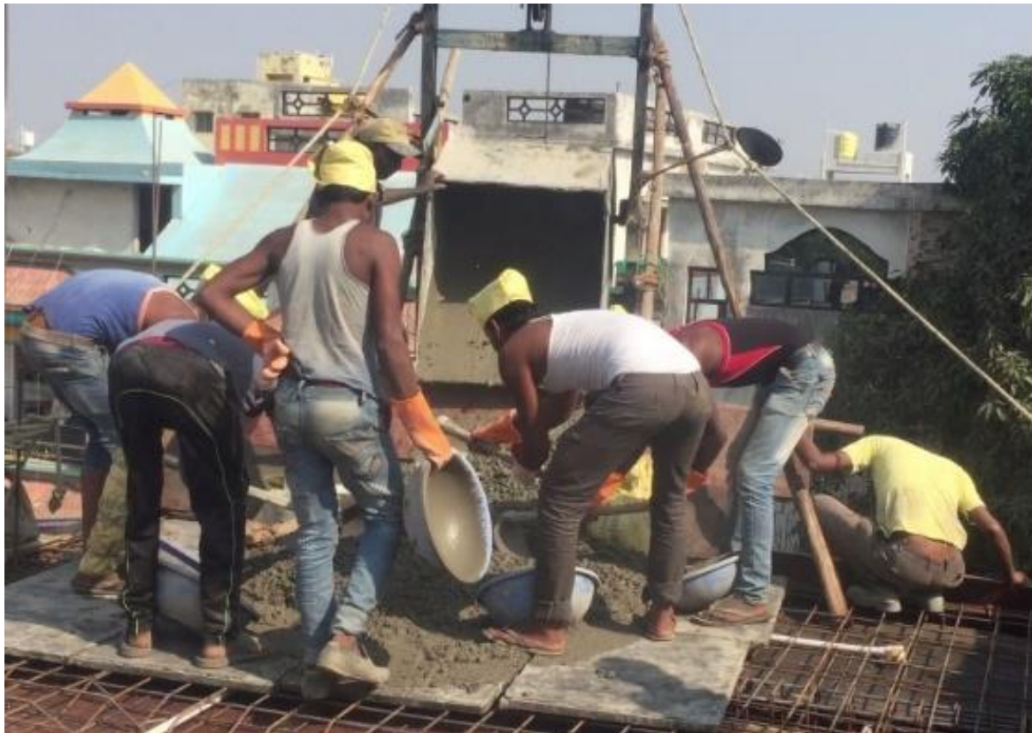
Figure (ii) Laborers collecting concrete in the iron-pan
