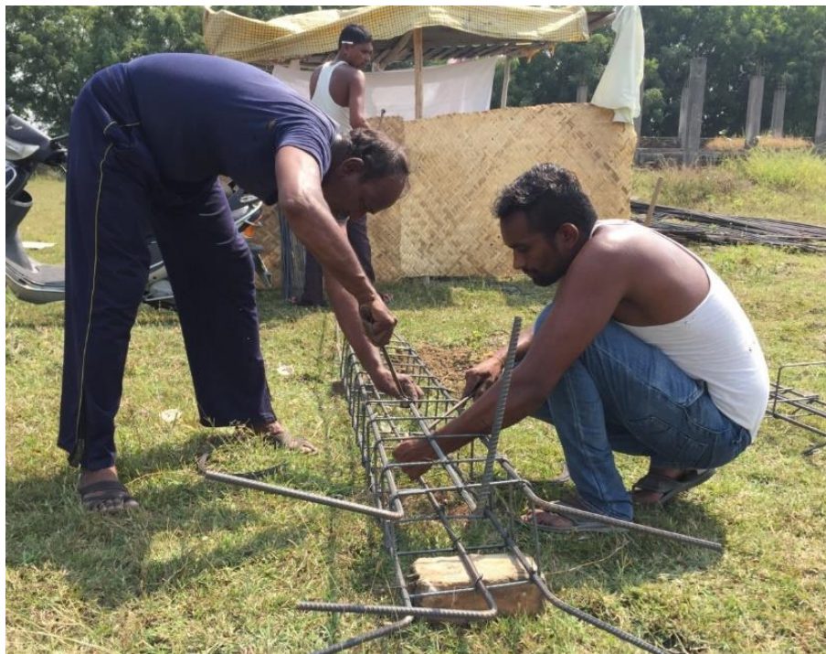
Figure (iv) Making of reinforcement / rebar steel cage for column (R4)
