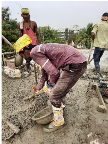
Figure (a): Collection of Concrete in the Iron-pan
