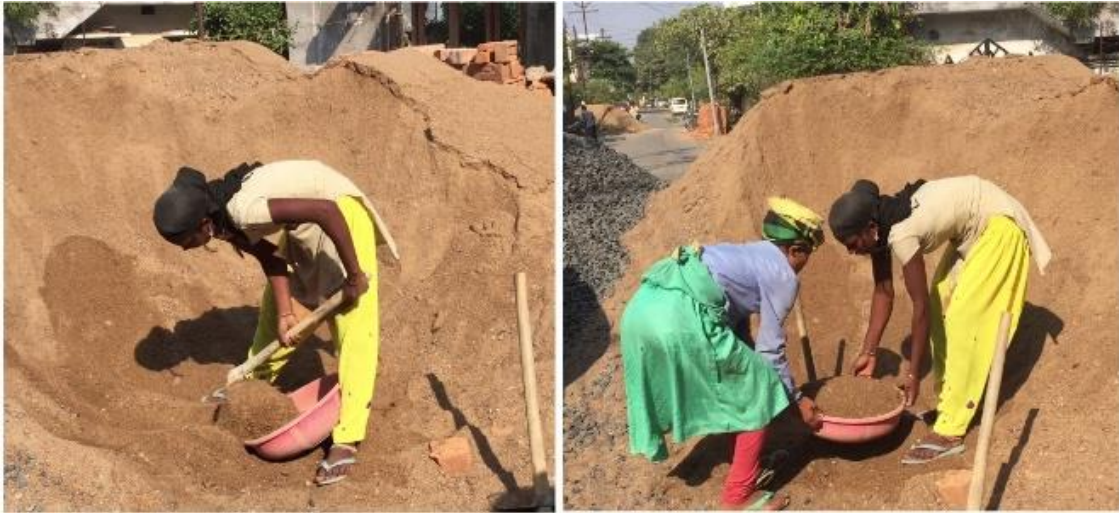
Figure (ii) Collecting, Lifting and Transportation of Sand
