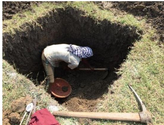
Figure (ii): Labourer performing collection of soil in Iron-pan (Job-2)
