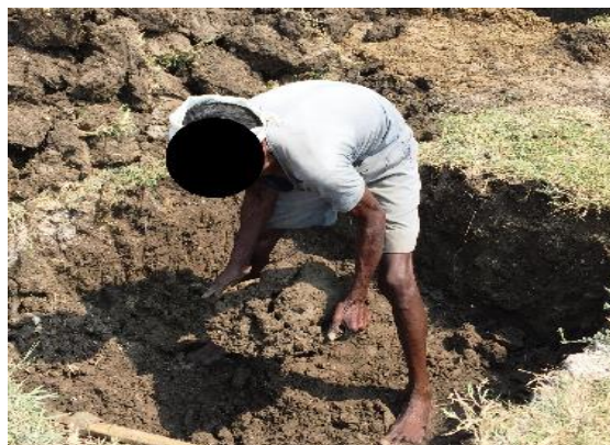
Figure (iii): Labourer performing lifting of Iron-pan (Job-3)
