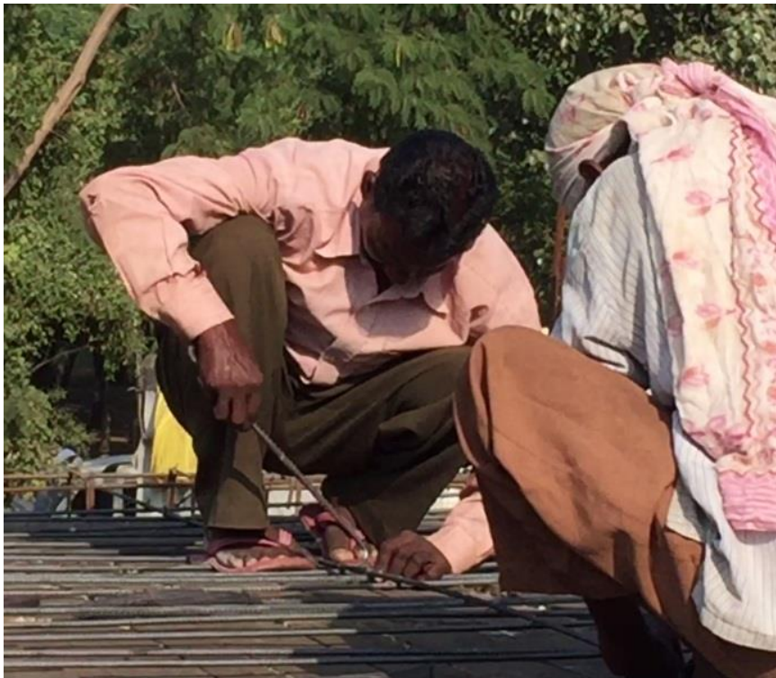
Figure (vi) Tying of Slab reinforcement / Rebar using iron wires (R6)
