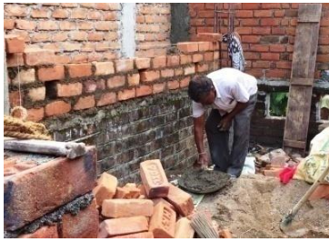
(a) Collect mortar from iron pan (BL-1)
