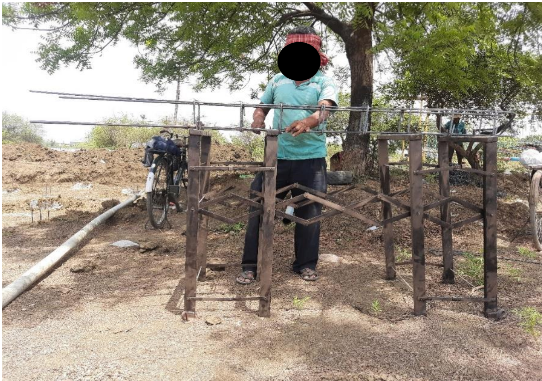
Figure 5.6 Rebar Cage tying with newly designed Foldable Multitasking Workable Platform
