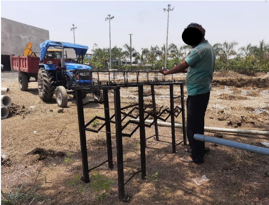
Figure 5.7 Rebar Cage tying with newly designed Foldable Multitasking Workable Platform
