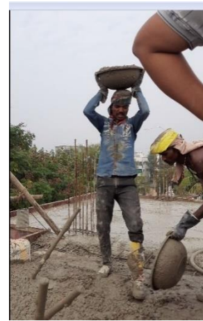
Figure (c): Lifting and holding Iron-Pan on head
