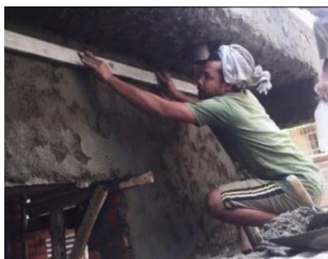
(g) Level / plain the mortar (for outside plastering) (PL-7)
