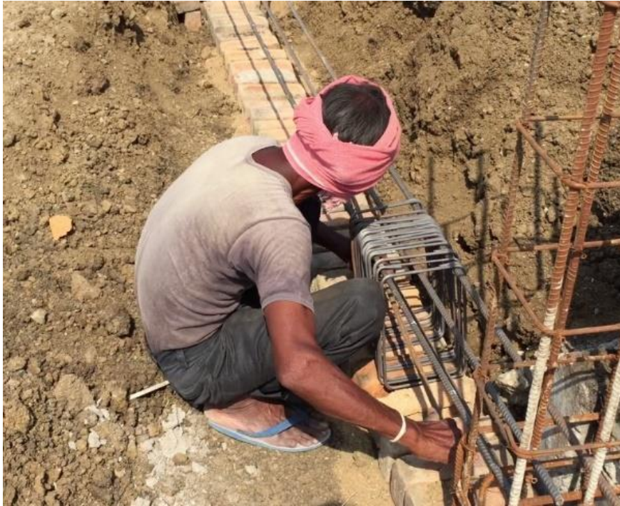
Figure (v) Tying stirrups in plinth and beam (R5)
