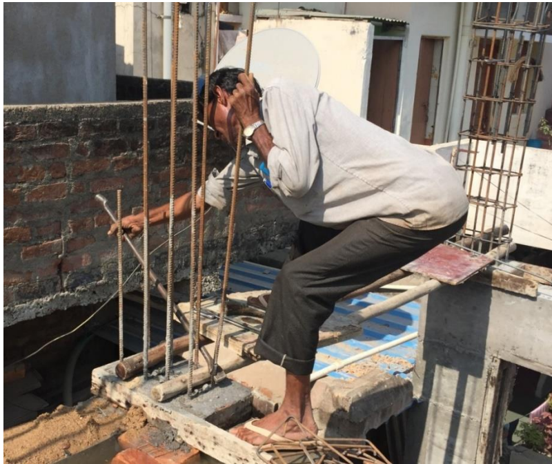
Figure (vii) Straightening of column rebar for extension of column (R7)
