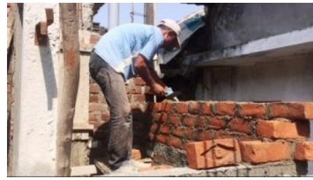
(b) laying of mortar bed (BL-2)
