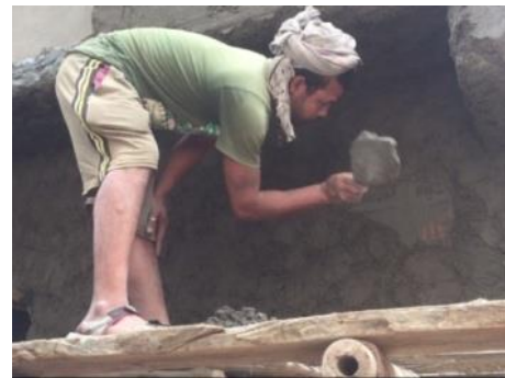
(f) Applying mortar on wall (for outside plastering) (PL-6)
