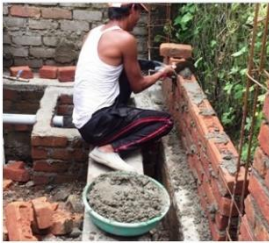
(c) Filling bricks gap(BL-3)
