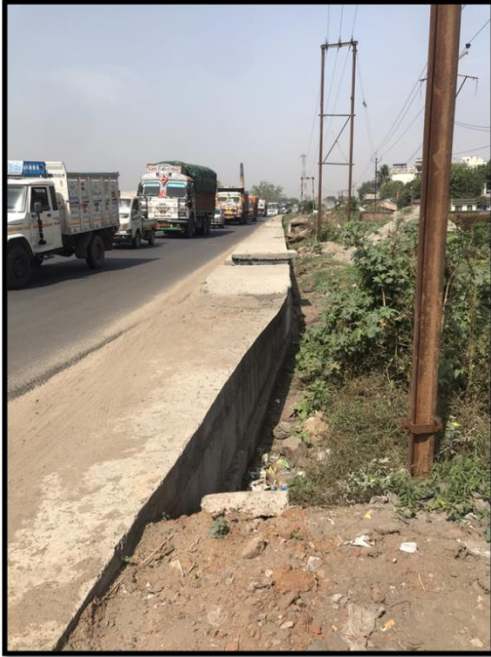
Photo.5.3.22 A and B Construction of High Drain at Bypass Road and Condition of Adjacent Drains adjacent to Ward No. 13
