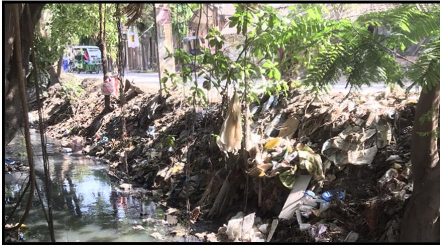
Photo.5.3.18. Condition of High Drain near Kalna Gate Ward No.12
