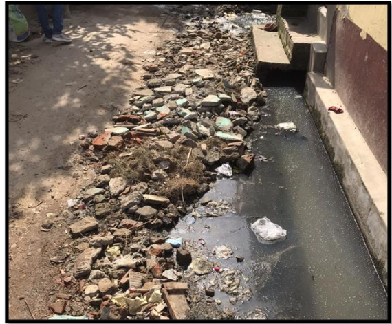
Photo.5.3.15 and 16 where the roads level off the drainages
