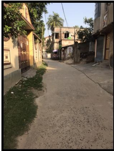
Photo.5.3.8. No Drainage on either side of the road
