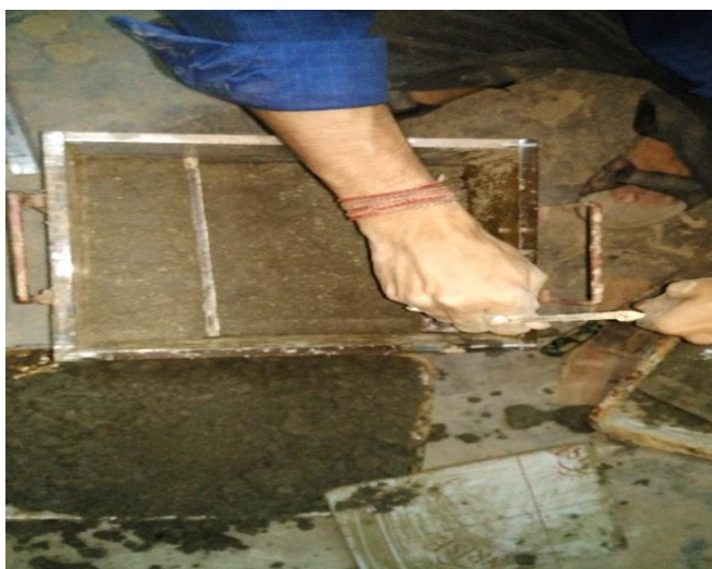
Fig. 4.12 Stage-3, Construction of Slope
