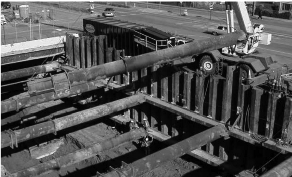
Figure 1 Sheet Pile Retaining Wall (Q. No. 3)
